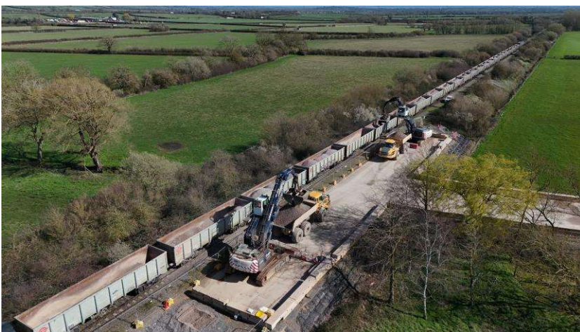
Pictured: Quainton Railhead – freight train material being unloaded for use across EKFB construction sites. March 2026
