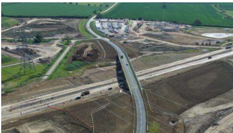
Pictured: Edgcott Overbridge carrying the realignment of Shipton Lee Road, Quainton.
